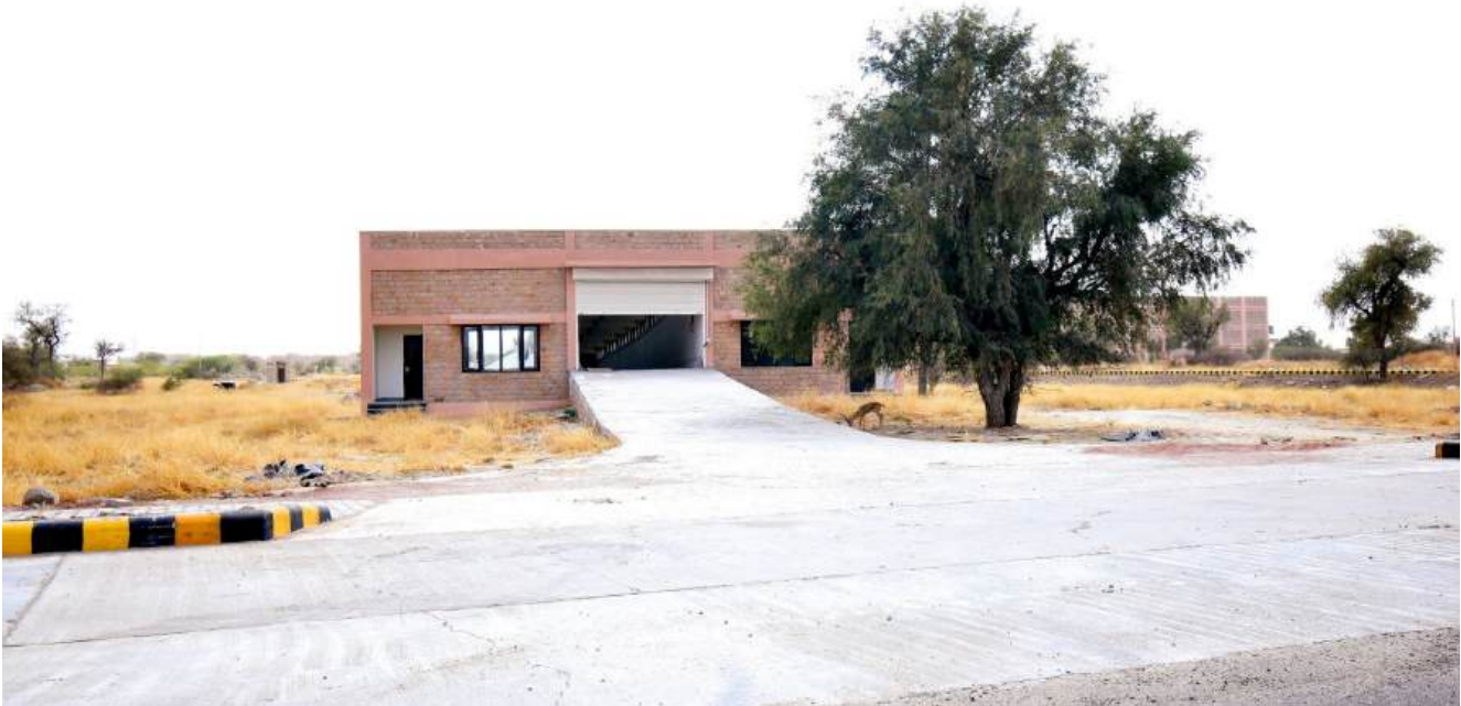
Utility Tunnel - Entrance Ramp
