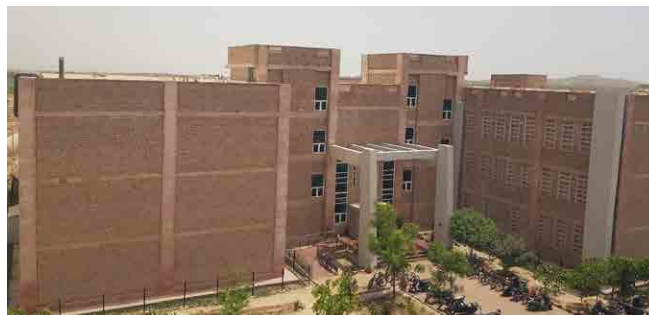
Metallurgical & Materials Engineering and Chemical Engineering Building
