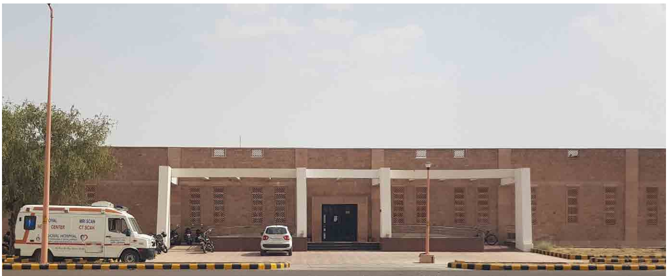
Primary Health Centre Building
