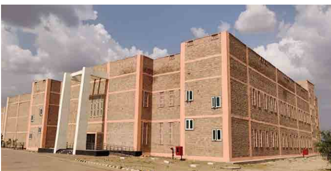
Civil and Infrastructure Engineering Building
