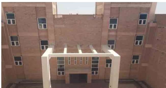
Computer Centre Building
